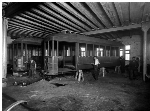
Trams of the city of Turku being renovated at the Fleminginkatu repair shop of Suomen Autoteollisuus, 1935. Photo: Olof Sundström. Source: Helsinki City Museum.
